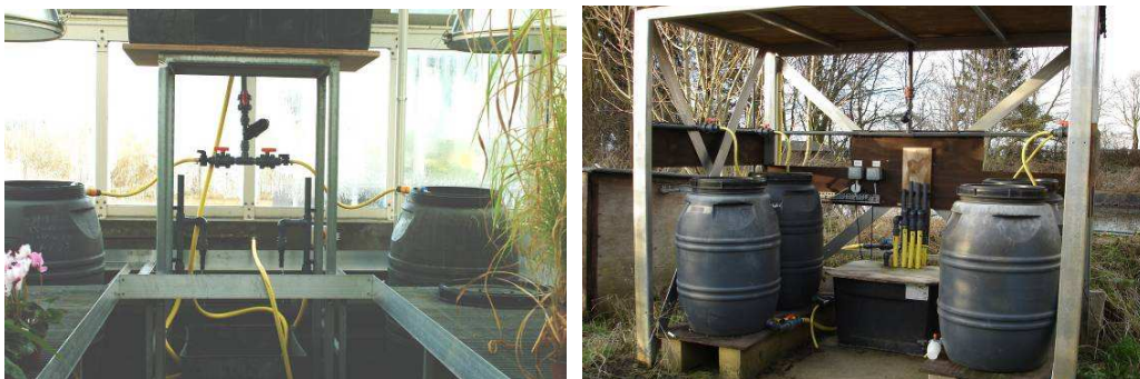
Figure 2. Slow sand filters held at CSL (left) and STC (right)
